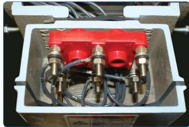
Oversized, gasketed IP-56 conduit box with lead separation gasket and conduit box cover gasket restricts moisture and contaminants from entering the motor.
